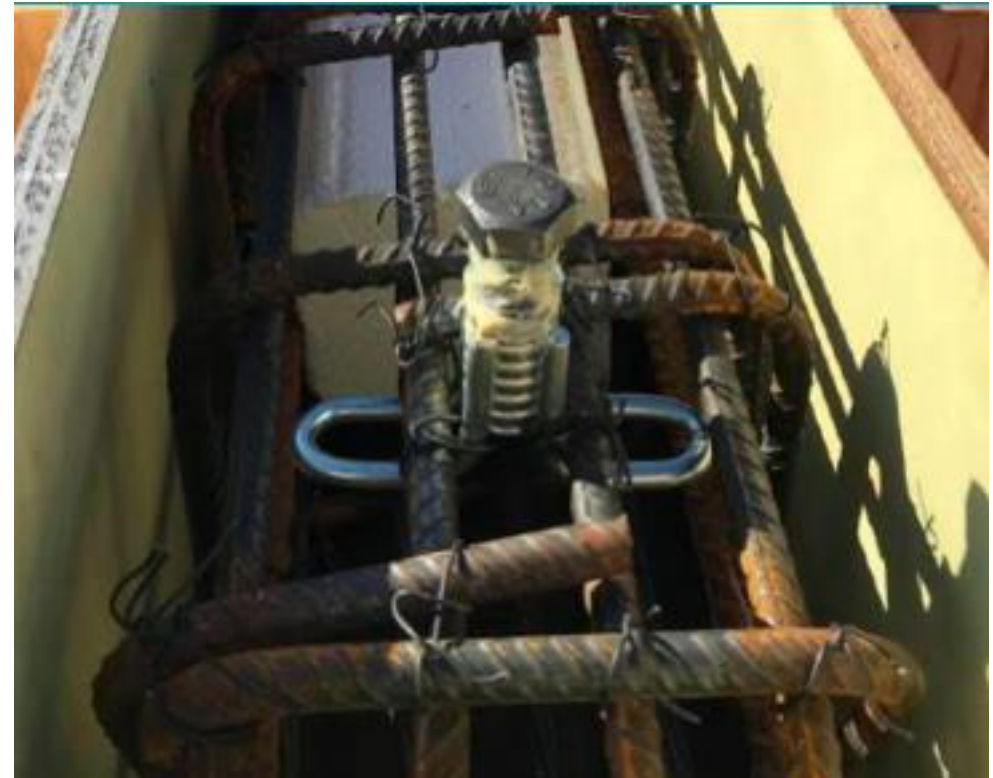
Figure 28. Last year's formwork
