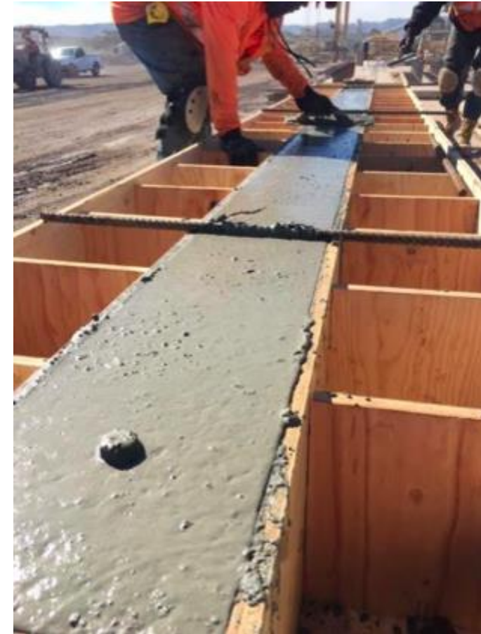
Figure 29. Last year's Screeding of Concrete
