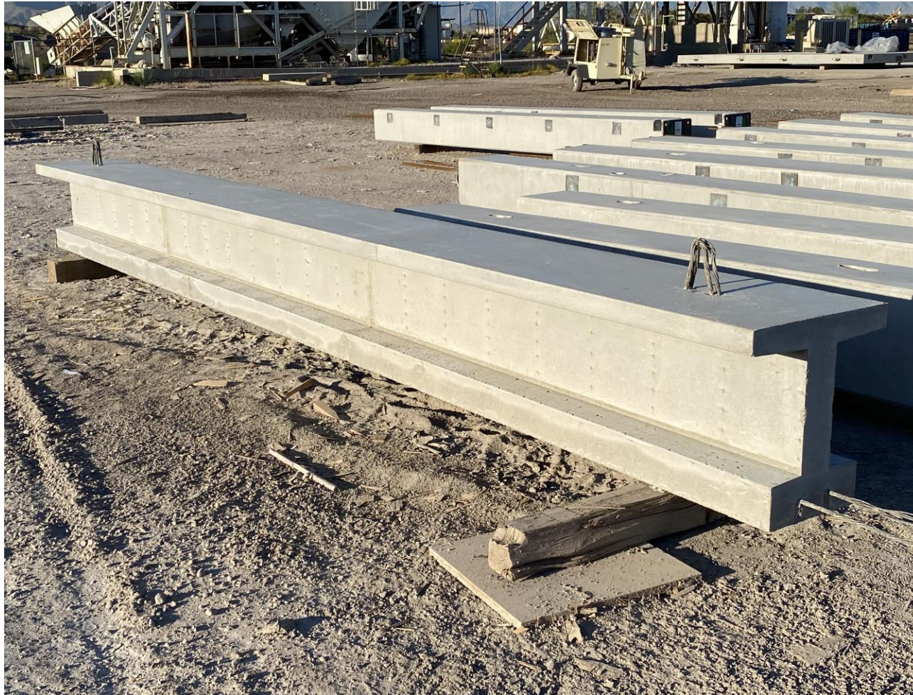
Figure 35. Beam at TPAC facility
